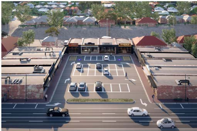
Before: Underutilised land limits opportunities for more homes, green spaces and vibrant communities.
