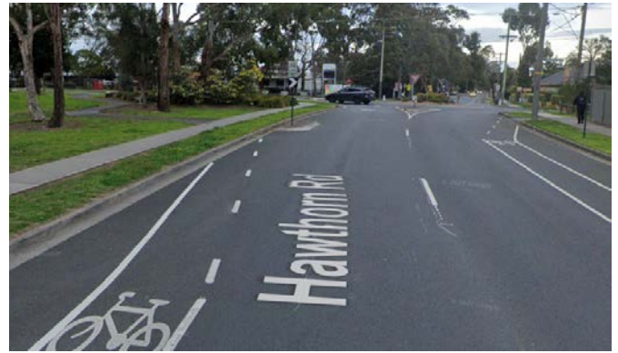
Figure 46 Issue: Bike Lane ends at obstacle, reducing space for cyclists when approaching the round-a-bout
