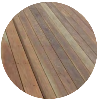
Decking on Pedestals Timber decking (Podium levels)
