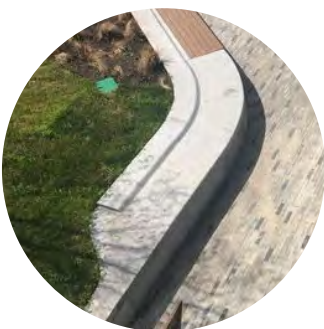
Concrete Walls Seating edges / Terraces
