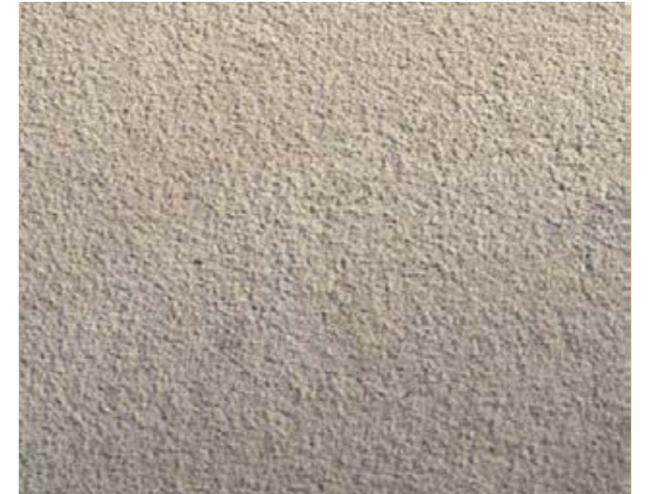
Lightly exposed aggregate concrete Source: AECOM
