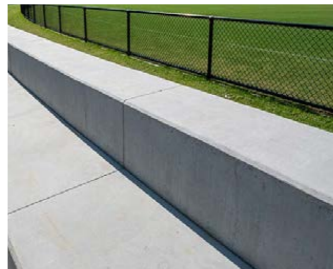
Concrete terrace seating Source: Concretum
