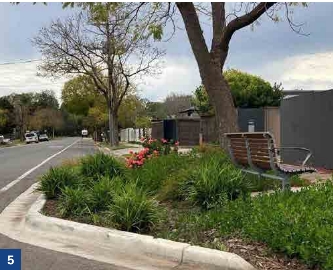
5 Street outkerb WSUD and tree planting - Lansdown Terrace Source: Walkerville Council, 2012
