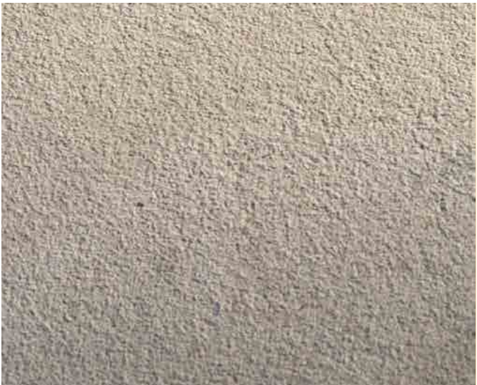
Lightly exposed aggregate concrete Source: AECOM
