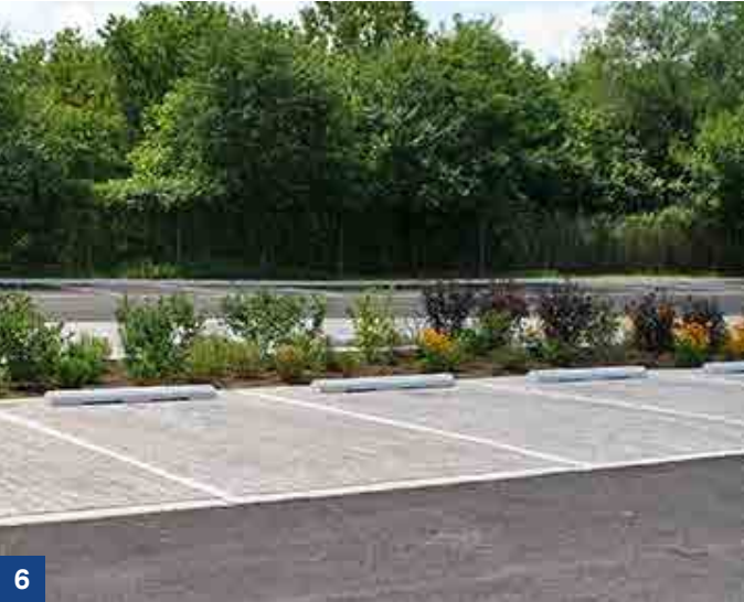
6 Permeable paving car parks - Curtin University Source: UDLA, 2021
