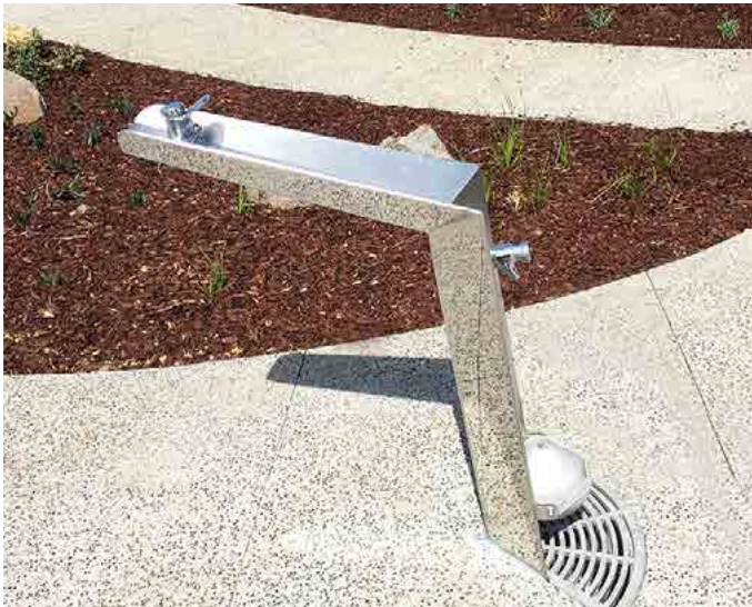
Accessible drinking fountain Source: Botton + Gardiner
