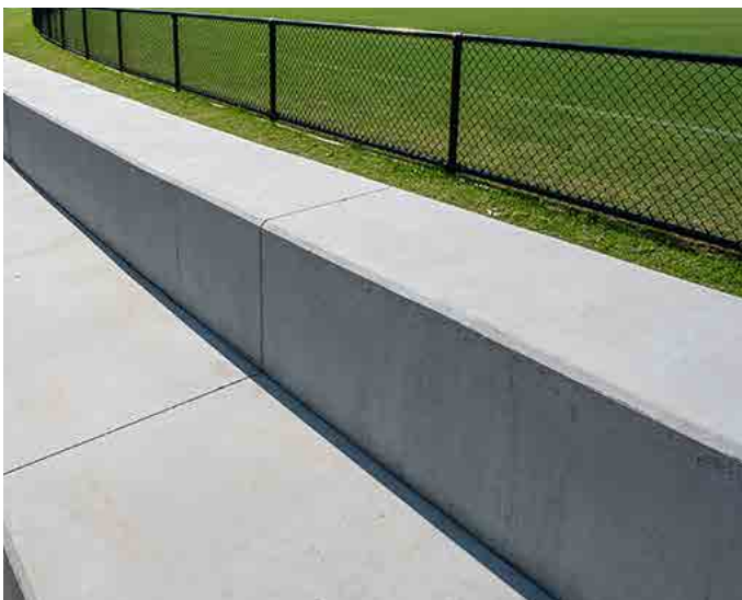
Concrete terrace seating Source: Concretum
